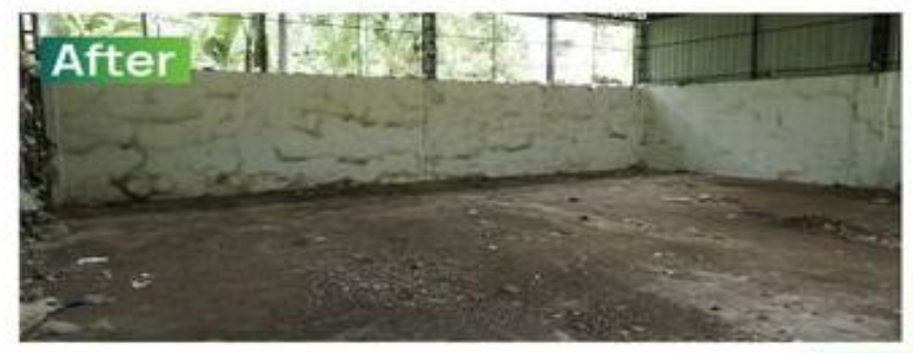
80 Tonnes of Waste Scientifically Processed & Disposed - Narikkuni Grama Panchayat -
